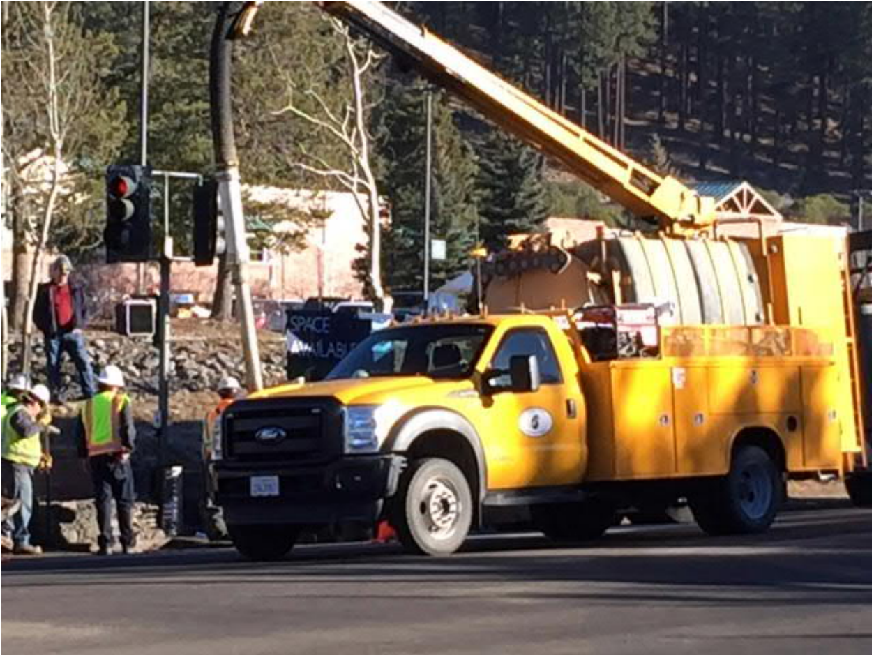
Water Crew repairing water main
