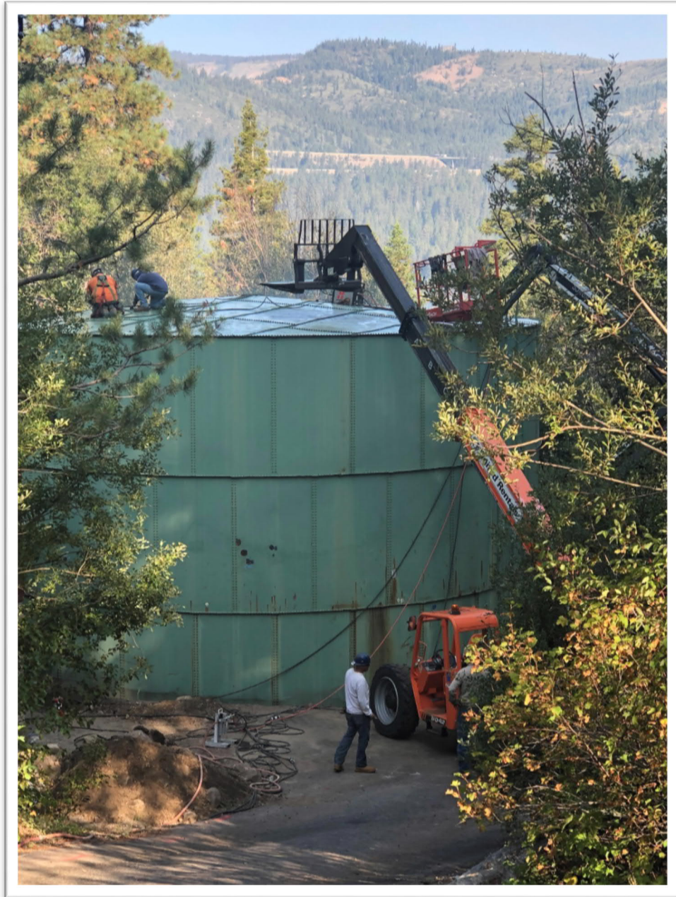
Deconstruction of Red Mountain Tank – Fall 2020
