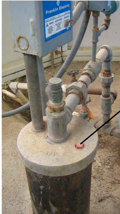
Photo: A domestic well showing the well casing, cover, and conveyance system. The well is located inside a shed with a concrete floor.
